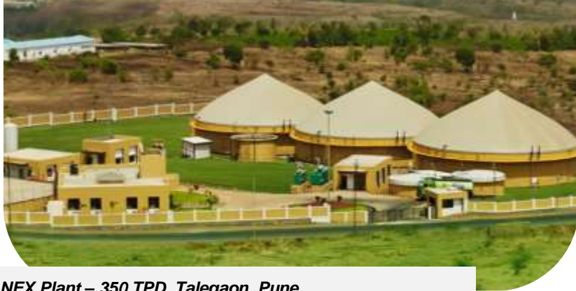
NEX Plant – 350 TPD, Talegaon, Pune
